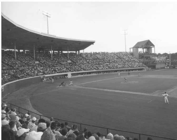
Current Technology® TransGuard® protects McCoy Stadium from harmful electrical surges.
