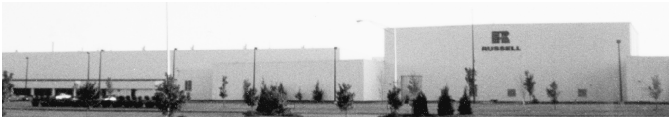
Russell Corp. Coosa River Plant
